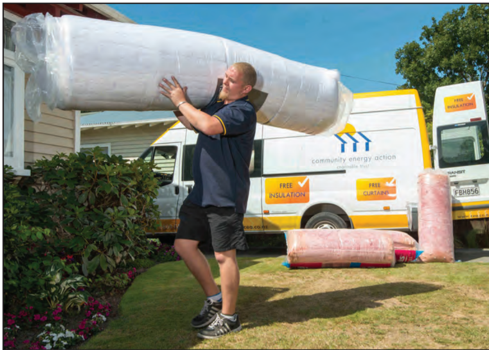
An installer from Community Energy Action on the job.
